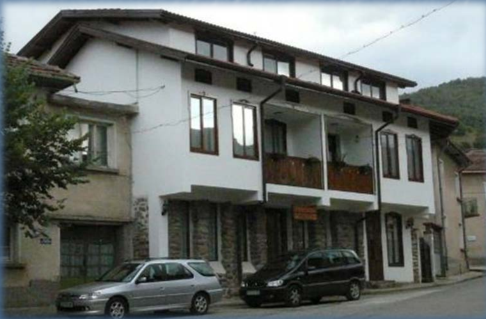
Guest house Torlatsite, Chiprovtsi
