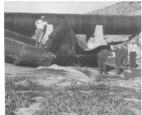
Los Angeles Aqueduct dynamited - 1927
